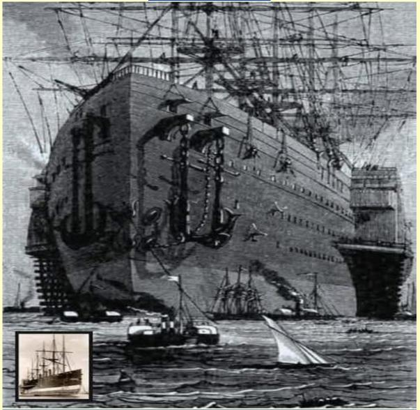
SS Great Eastern, designed by Isambard Kingdom Brunel, was the largest ship ever built when it was completed in 1858. It could transport up to 4,000 passengers from England to Australia without refueling, making it a technical masterpiece of its time. The SS Great Eastern was equipped with sails, paddle wheels and a screw drive, marking a turning point in shipbuilding. Her length of 211 meters and her double hull were revolutionary features that were later adopted in shipbuilding.
